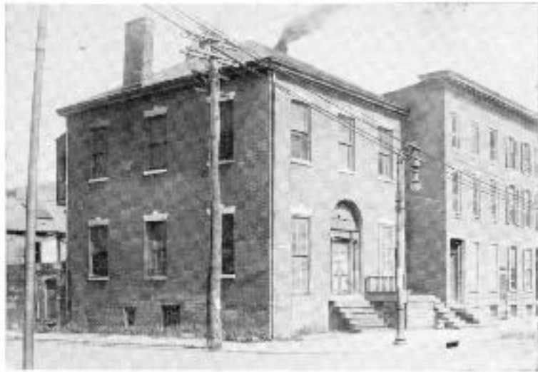
THE STATE BANK BUILDING. Before it was demolished in 1921.
