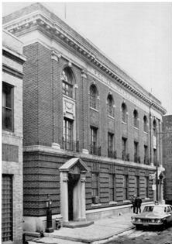
HEADQUARTERS AND FIRST PRECINCT STATION In 1964.
