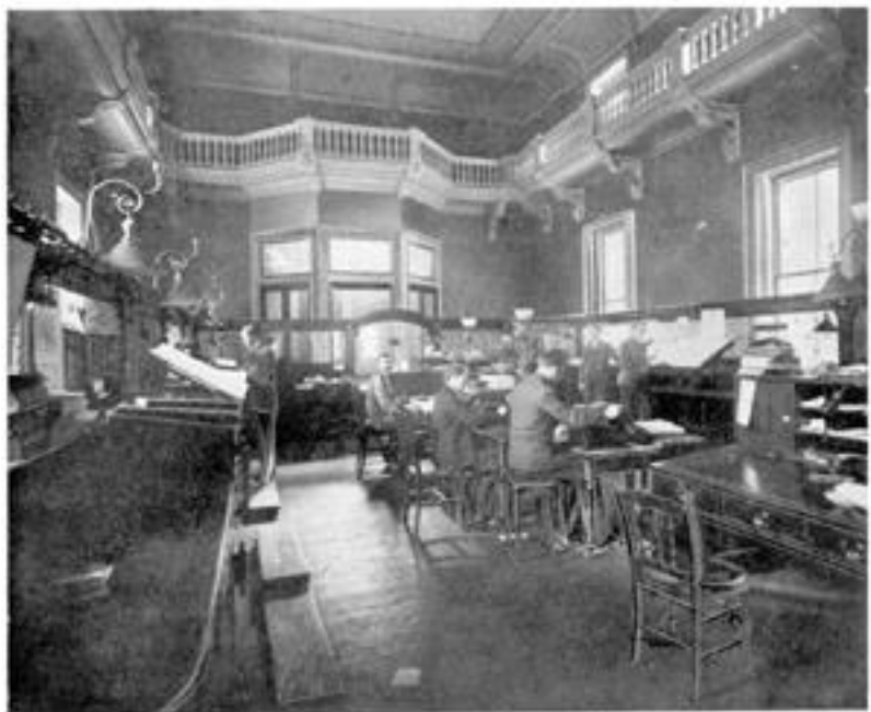
INTERIOR VIEW OF OLD TRENTON BANKING COMPANY BUILDING
