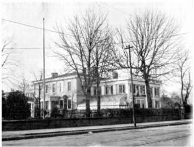
THE WILLIAM TRENT HOUSE Before 1936 restoration.
