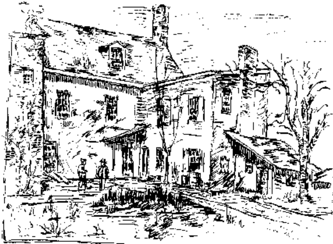
REAR VIEW OF THE BREARLEY HOUSE
