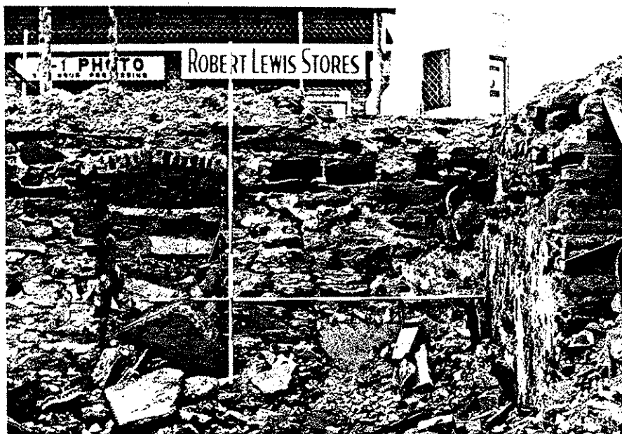
Plate D.13. 2 North Warren Street: view of the southwest corner foundation, looking south, showing blocked opening to possible vault beneath sidewalk; scale in feet (Photographer: Lynn Rakos, November 1987).
