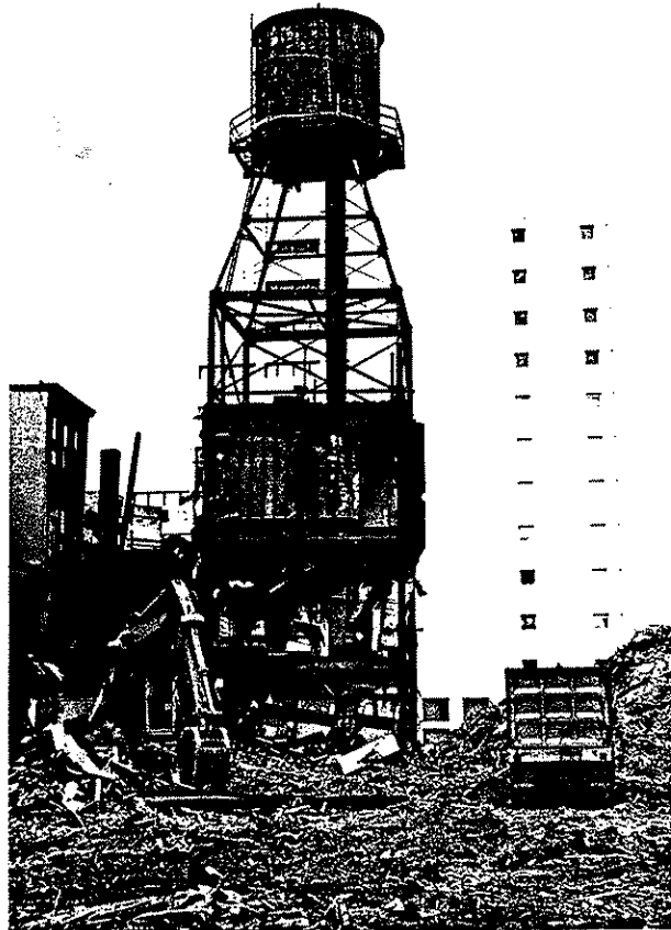
Plate D.5. View of the Dunhams water tower, looking west, taken during the demolition of the block (Photographer: Steven Kaplan, November 1987).
