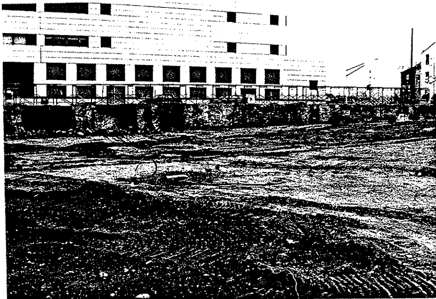
Plate D.12. General view looking northwest following demolition and excavation of the Dunhams Block; foundations of structures fronting on North Warren Street are visible at center of photograph (Photographer: Lynn Rakos, November 1987).
