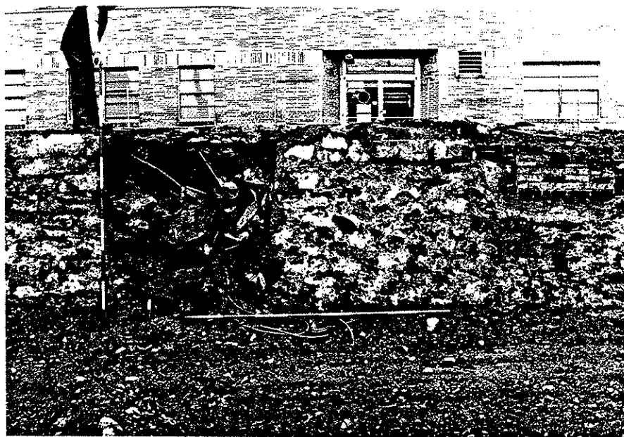
Plate D.6. View looking north, at the north foundation of the mid-1850s wing of the Trenton House; East Hanover Street in background; scale in feet (Photographer: Lynn Rakos, November 1987).
