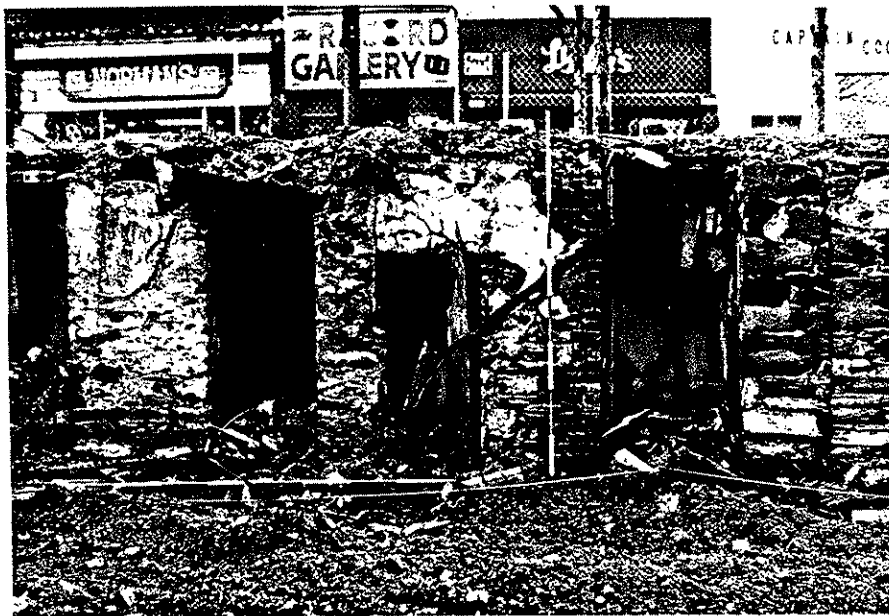
Plate D.14. 8 East State Street: view looking south at south foundation; small doorway in center leads into a stone lined, brick-arched vault located beneath sidewalk; scale in feet (Photographer: Lynn Rakos, November 1987).
