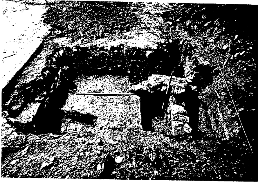
Plate 6.21. 14 North Warren Street, Alley Excavation Unit: general view looking west showing series of 19th and possible late 18th century stone walls; scale in feet (Photographer: Richard Hunter, May 1987).
