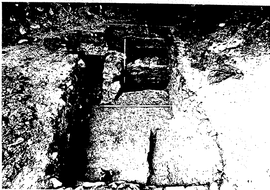
Plate 6.20. 14 North Warren Street, Alley Excavation Unit: general view looking north showing series of 19th and possible late 18th century stone walls; scale in feet (Photographer: Richard Hunter, May 1987).
